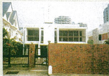
The house before reconstruction.
